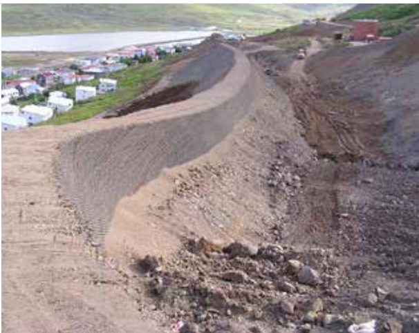
Figure 3: Catching dam in construction: the steep top section is made of geocells
