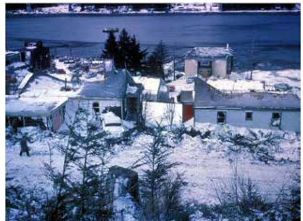
Figure 4: View of Behrends Avenue with Gastineau Channel in the background after the 1962 avalanche: collapsed roofs because of overpressure and impacts of trees. The back-walls are not damaged
