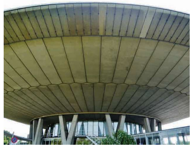
Figure 3: Prefab ring-elements, including thermocouples in the outer ring
