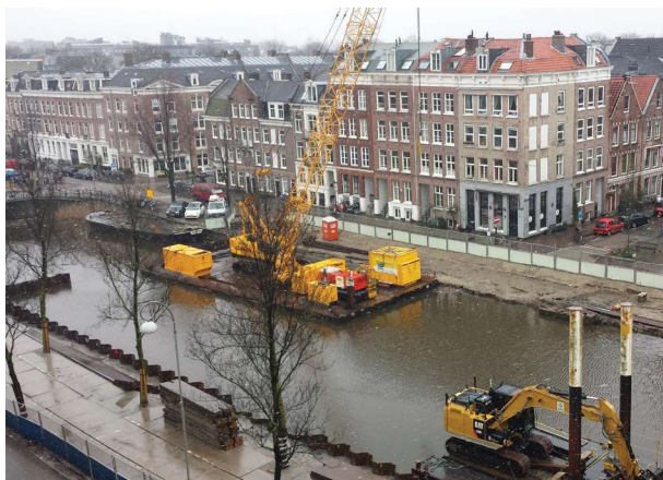
Figure 1: Installation of sheet pile walls at the Ruysdaelkade
