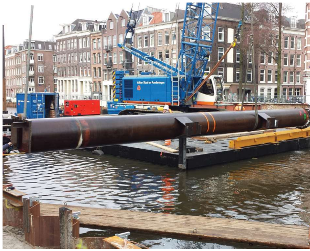
Figure 2: Placing the struts
