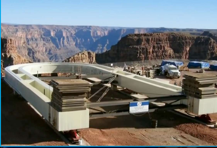
Skywalk during construction
