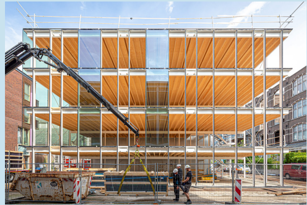
Figure 3: Glass facades installation
