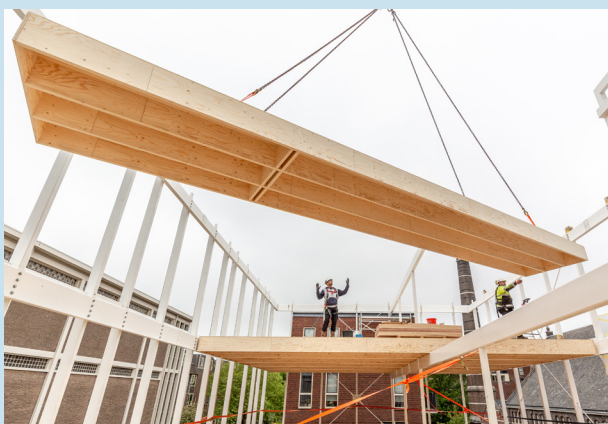
Figure 2: Wooden floors installation
