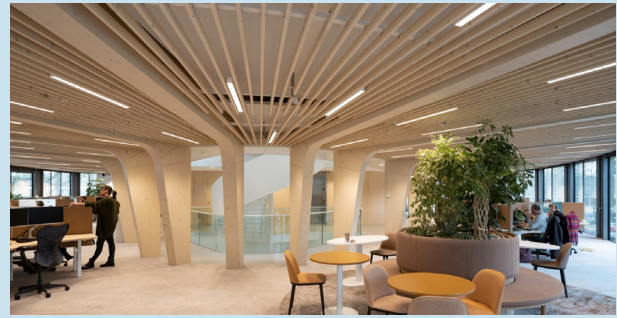
Figure 3: Curved timber elements
