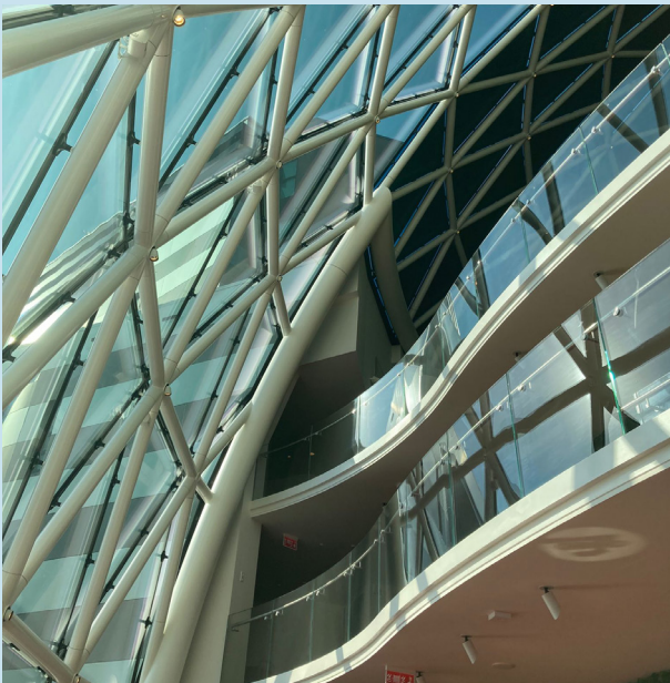
Figure 3: Edge beam around connection to theatre tower
