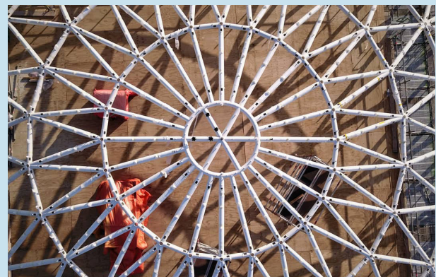
Figure 5: Final ring installed at the top of the dome
