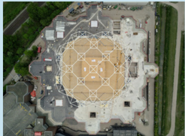
Figure 8: The dome under construction
