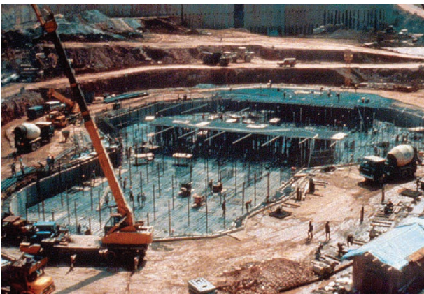
Figure 1: Construction of the massive foundation of Tower 1
