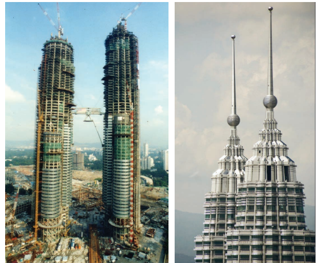
Figure 4: The finishing touch of the Petronas Towers
