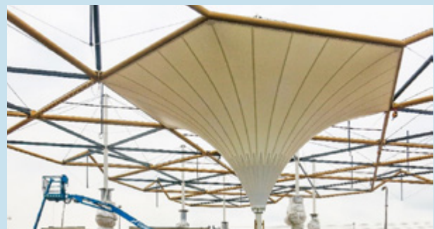
Figure 1: Construction of the bus station
