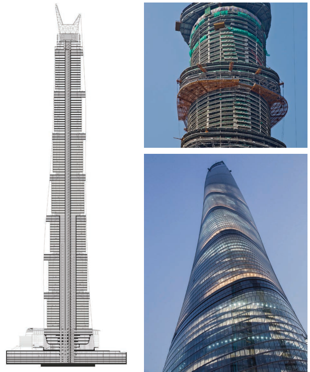
Figure 8: The tower section, construction, and skin during/after construction
