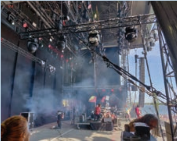
Figure 2: Stability bracing connection in bottom right at best kept secret mainstage
