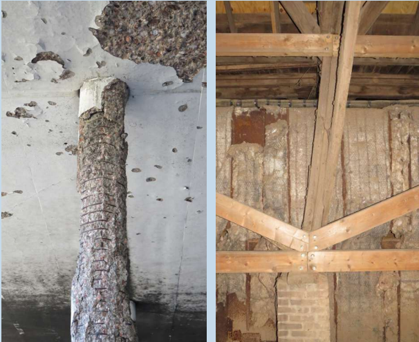
Figure 2: Damage due to fire in Kantinegebouw Enka, Ede (left), Deformed timber structure in Steenfabriek, Elden (right)
