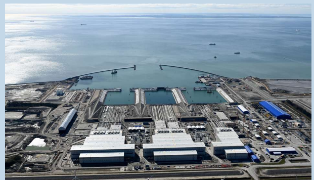
Figure 2: Working harbour on Lolland, at the bottom of the picture the three halls of the tunnel element production facility including the basins (Photo: Femern A/S)
