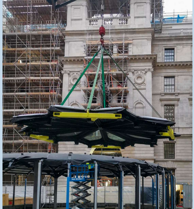
Figure 4: Assembly on-site (Photo: Octatube)
