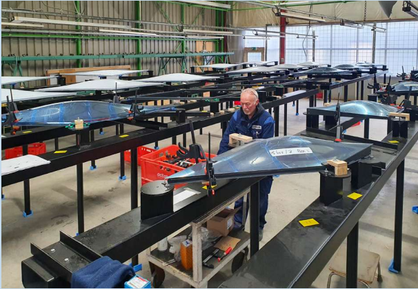
Figure 2: Manufacturing of the roof panels (Photo: Octatube)
