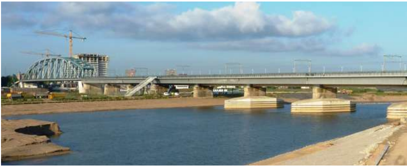
Figure 4: Reinforced piers railroad bridge
