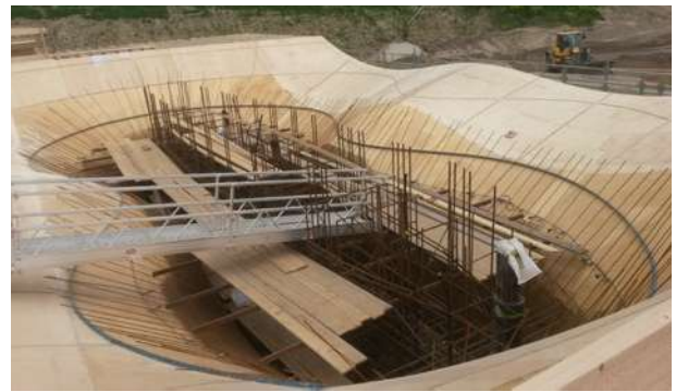
Figure 6: i-Lent formwork for the extended 'Waalbrug'
