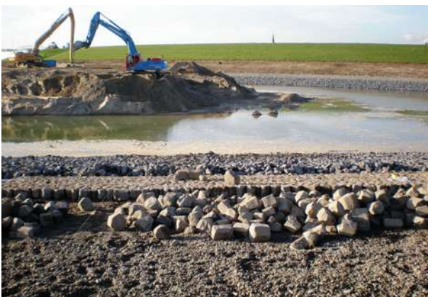
Figure 5: Construction of the new dike
