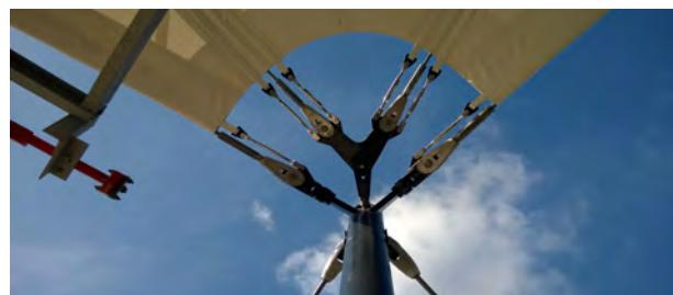
Figure 5: Connection of the fabric to the edge column
