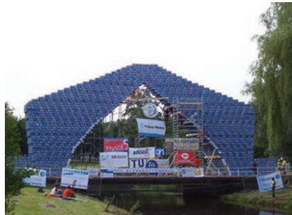
2005 - Daily construction progress of Eindhoven's first Beer Crate Bridge
