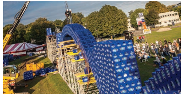
Figure 3: Beer Crate Bridge, 2012
