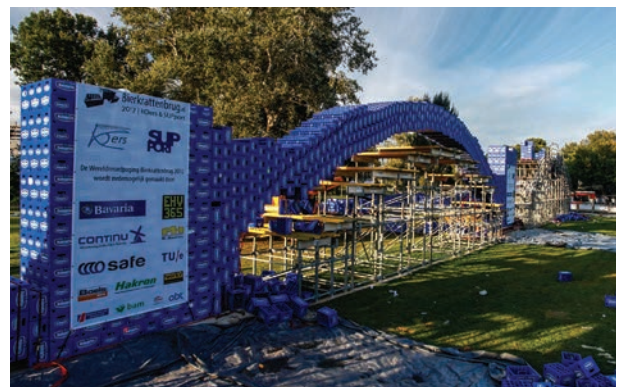
Figure 1: Beer Crate Bridge, 2012
