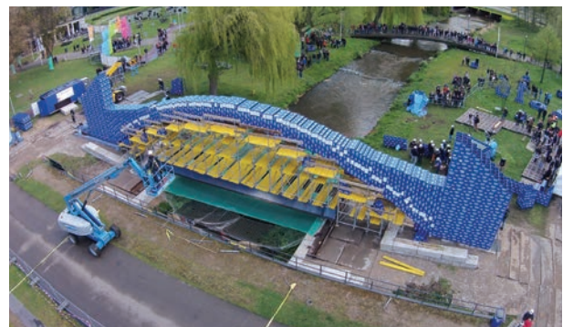
Figure 1: Drone overview of the Beer Crate Bridge, 2016
