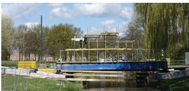
Figure 3: Supporting structure of the Beer Crate Bridge, 2016
