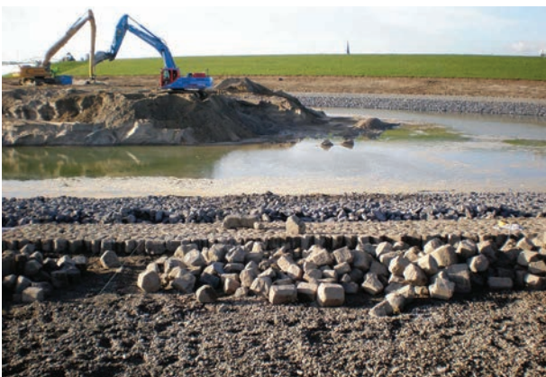
Figure 5: Construction of the new dike
