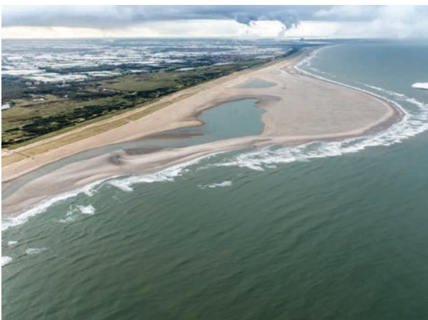
Figure 4: Overview of the Sand Motor (2012)
