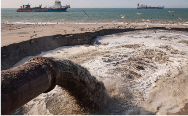
Figure 2: Construction of the Sand Motor (left and right)
