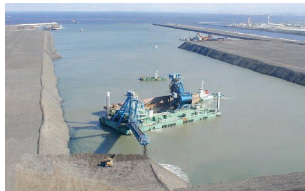
Figure 1: Building the artificial island
