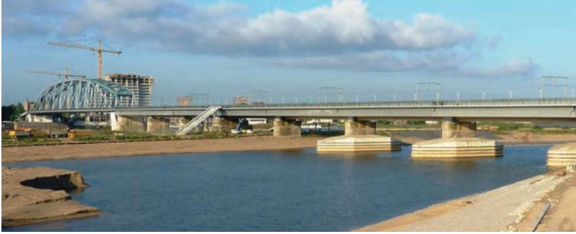
Figure 4: Reinforced piers railroad bridge
