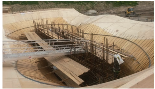
Figure 6: i-Lent formwork for the extended 'Waalbrug'
