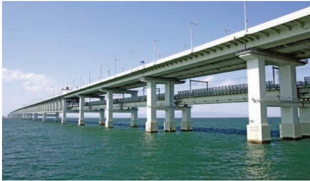
Figure 2: The Sky Gate Bridge
