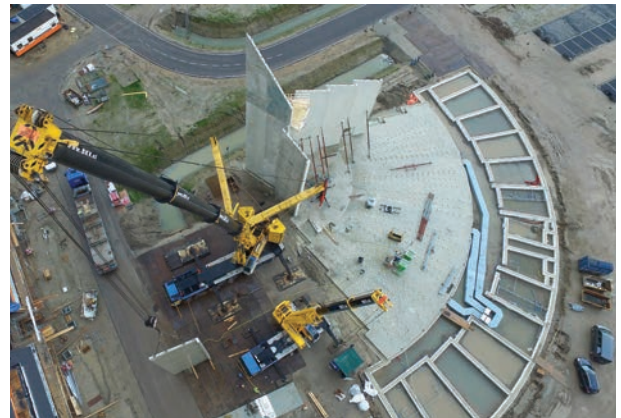
Figure 2: Foundation church. Floors and foundation by B-smart foundation
