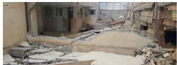
Figure 6: No buttressing of boundary (yard) walls
