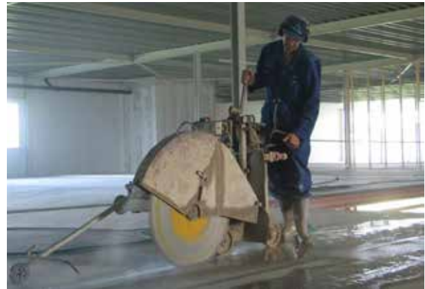
Figure 1: Sawing a concrete floor (Wijma bv)
