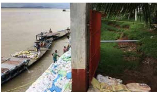
Figure 4: 'Low-tech' temporarily embankment protection after the first flood and monsoon on June 11 th and 12 th
