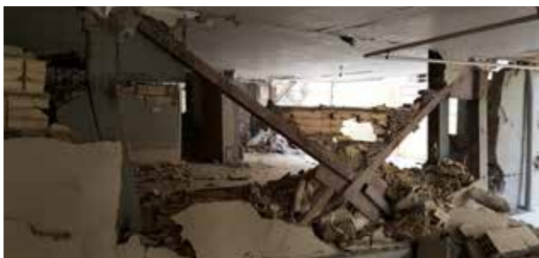
Figure 5: Improper connection of wall and structural elements
