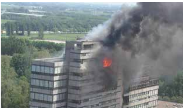
Figure 2: TU Delft department of Building and Architecture on fire; building completely demolished by a travelling compartment fire
