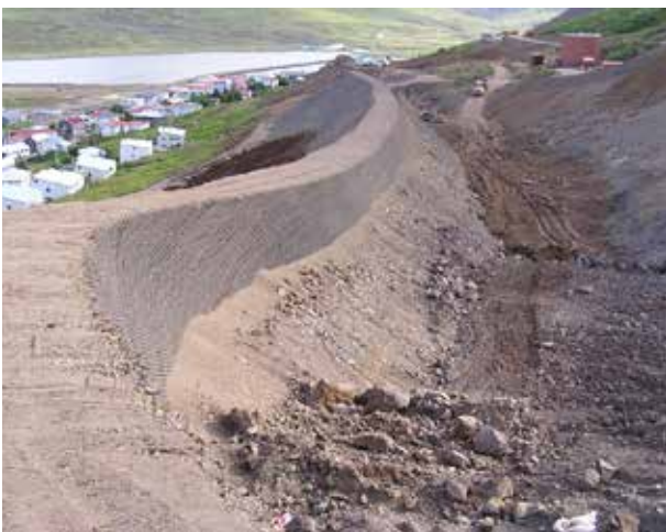
Figure 3: Catching dam in construction: the steep top section is made of geocells
