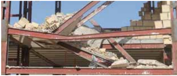
Figure 3: Collapsed stairs due to poor design
