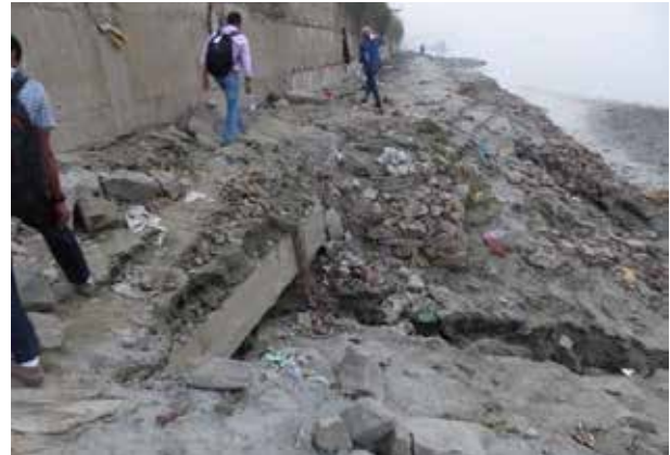
Figure 5: Eroded embankment and protection structures flushed away in 2017
