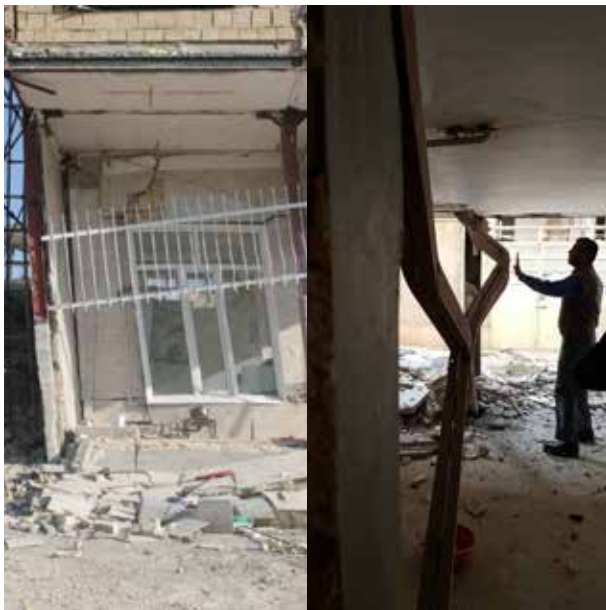
Figure 1: Soft story on ground floor (left) and global buckling of braces (right)
