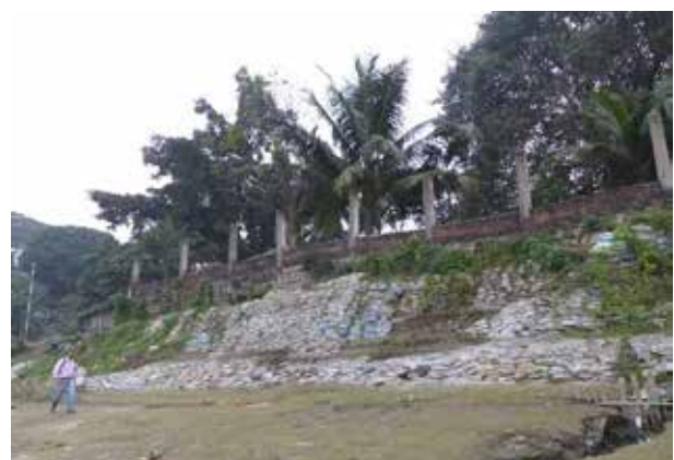
Figure 6: 'Low-tech' temporarily embankment protection after the first flood and monsoon on June 11 th and 12 th
