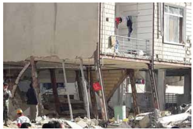
Figure 2: Inappropriate performance of structures with two different lateral displacement resisting systems in two orthogonal directions
