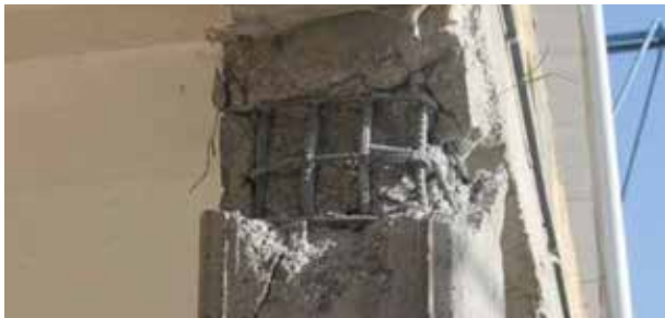
Figure 4: Lack of transverse rebars
