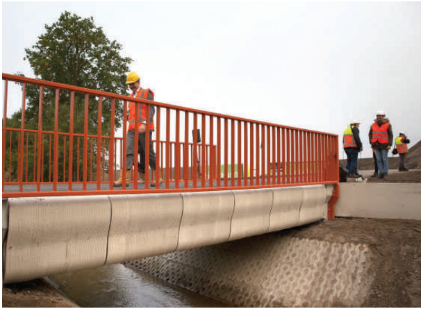
Figure 2: First 3D printed bridge in Gemert, the Netherlands
