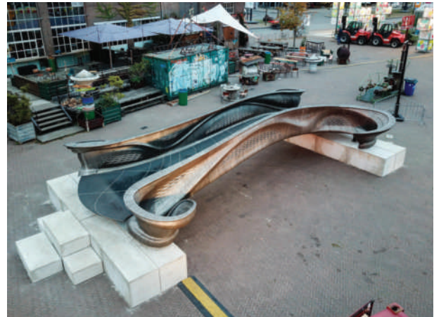
Figure 2: The printed stainless steel bridge by MX3D at the Dutch Design Week 2018 in Eindhoven
