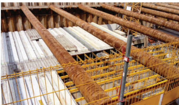
Figure 2: Slab floor with EPS weight reduction
