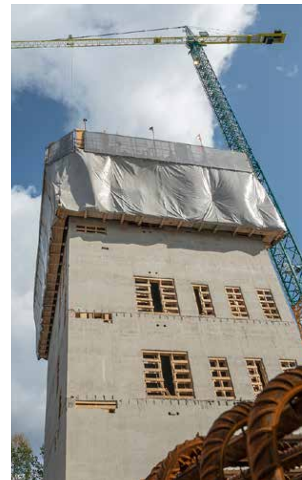
Figure 1: Slipform system at European Medicines Agency (EMA) (Photo: Rob Acket - Piktsjers)
