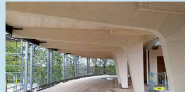
Figure 2: Standard floor with timber rafters
