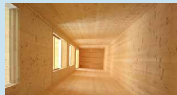
Figure 3: CLT-walls of the elevator
