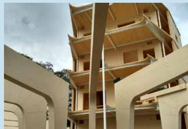
Figure 1: Timber cantilever rafters and core
