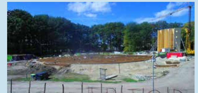
Figure 4: CLT-walls of the core of 4 building layers
