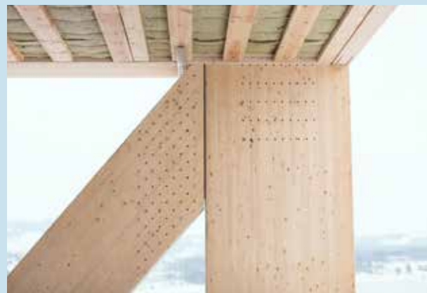
Figure 4: Detail Timber connection (photo Øivind Haug)
