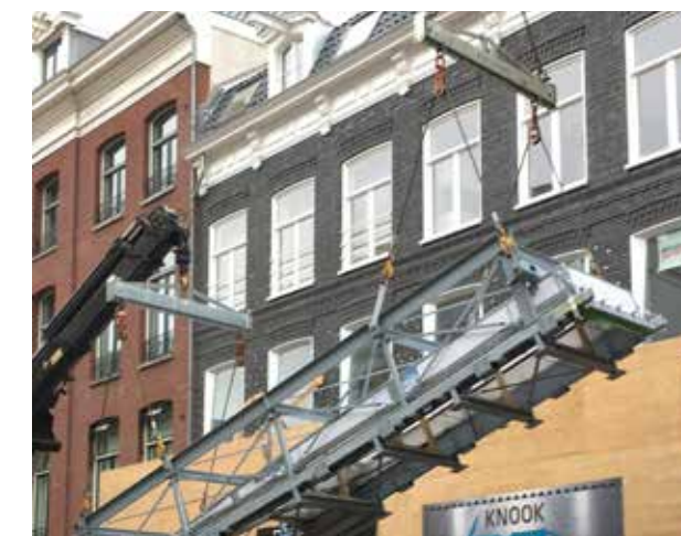
Figure 4: lifting the auxiliary frame
